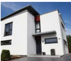
Vollheizung Full heating
