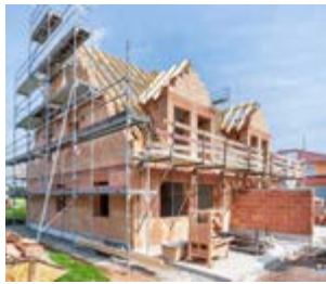
Neubau New building
